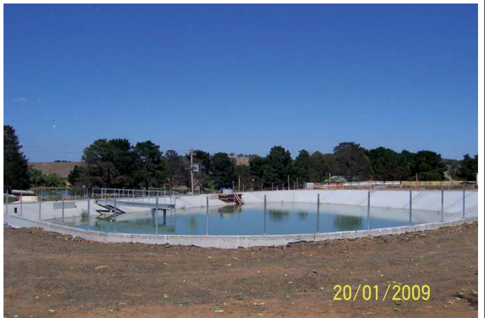
Sludge Lagoon No 3 - work significantly completed
