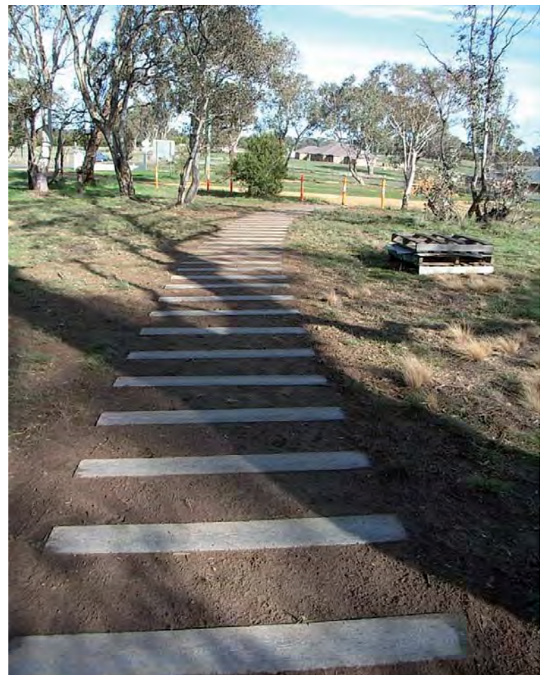
Concrete sleeper pathway under construction at Murrumbateman Cemetery
